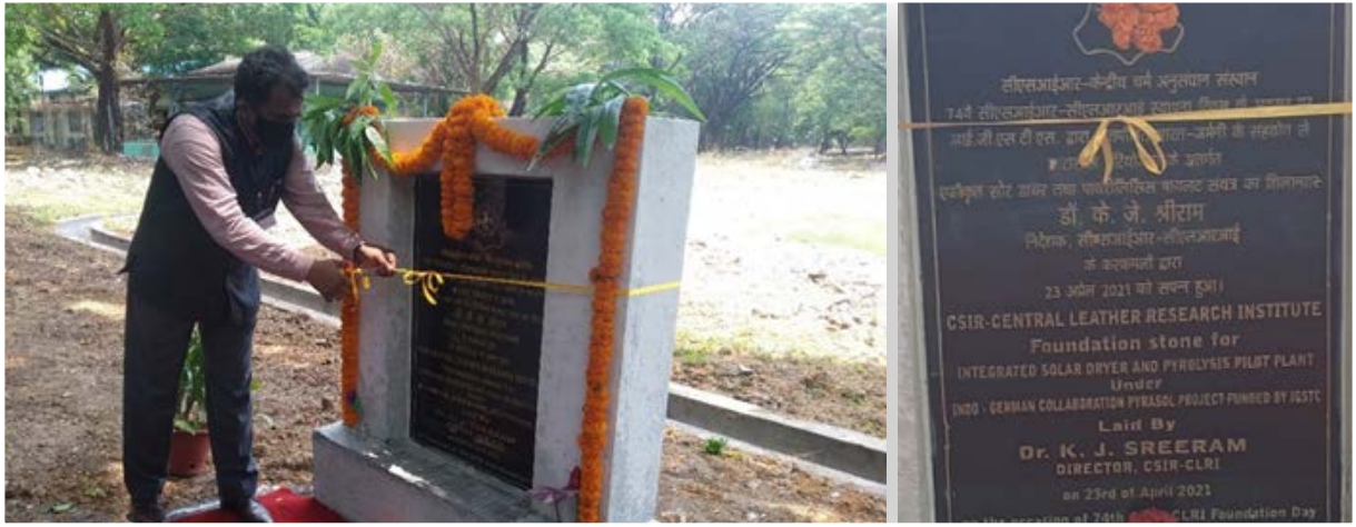
Dr K.J. Sreeram, Director, CSIR-CLRI inaugurating the foundation stone of integrated solar dryer and pyrolysis plant
